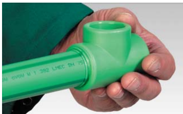
...putting the fitting in the right direction
