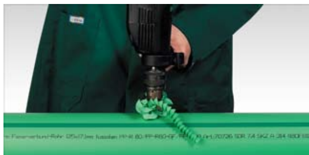
Drilling through the pipe wall
