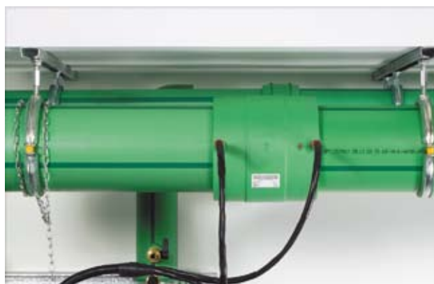
Adjust the socket diameter on the welding device. Start and control welding process. Keep the cooling time. Finished!
