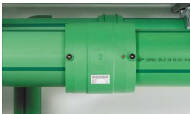
Push the second pipe - also peeled and cleaned - into the socket
