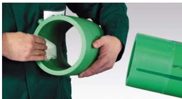
Clean the inner surface of the electrofusion socket
