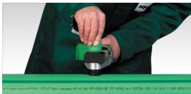
...heating-up of the pipe and fitting.
