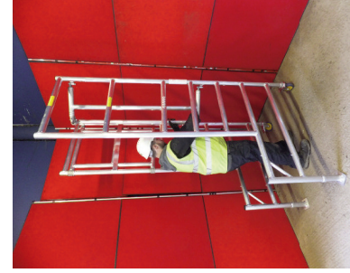
2. OPEN FRAMEWORK AND ENSURE MECHANISM IS LOCKED
