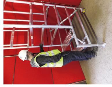
3. FIT TWO DIAGONALS AT REAR FOR STANDARD PODIUM WITH STEPS, AND THEN TWO CLIMBING BRACES FITTED ON TO VERTICALS AND RESTING ON SIDE BARS. FIT PLATFORM.
