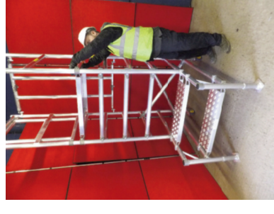
3. FIT TWO DIAGONALS AT REAR FOR STANDARD PODIUM WITH STEPS, AND THEN THREE CLIMBING BRACES FITTED ON TO VERTICALS AND RESTING ON SIDE BARS. FIT PLATFORM.
