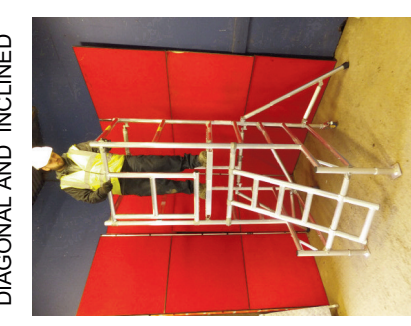
4. FOR PAS250 OPTION FIT ONE DIAGONAL AND INCLINED
