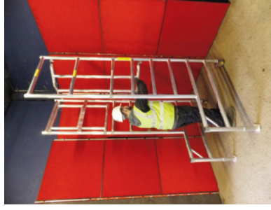
2. OPEN FRAMEWORK AND ENSURE MECHANISM IS LOCKED
