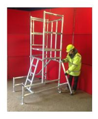
6) DEPLOY STABILISERS IN CORRECT POSITION
