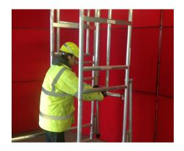
1) OPEN FRAME AND LOCK MECHANISM
