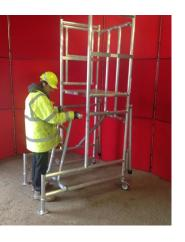
4) CLIP UPPER BRACE OF LADDER ABOVE RINGS ON VERTICALS WITH ASSEMBLED HOOKS ON TOP
