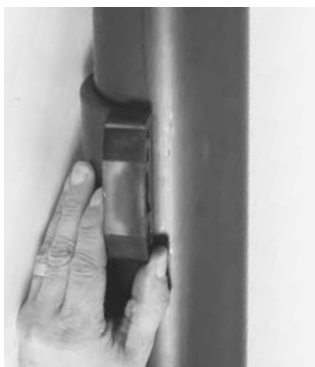
1. Position lower half of saddle around pipe.
